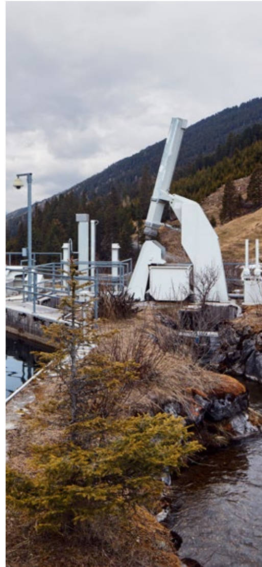
Swarovski hydropower water inlet, Wattens, Austria
